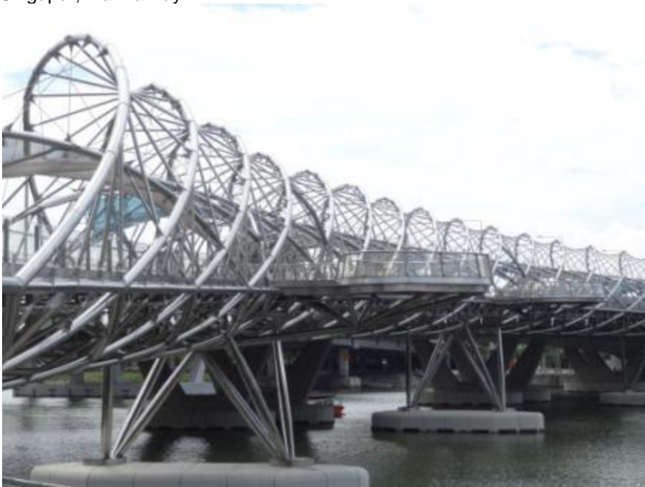
Singapur, Helix Bridge
